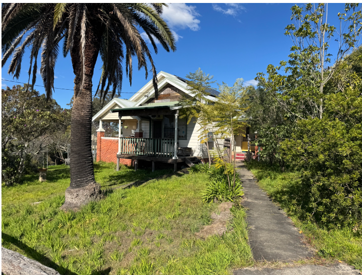
Figure 5 The existing dwelling viewed from Myles Street.
