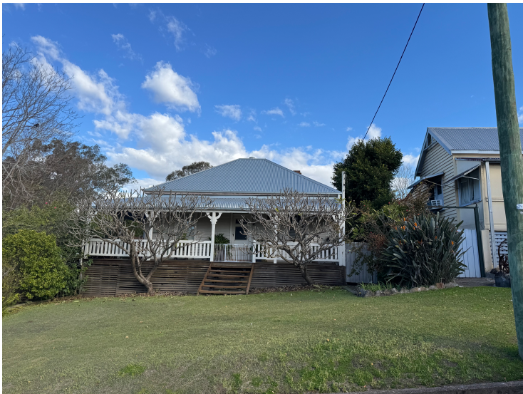
Figure 7 The dwelling at #34 Myles Street.
