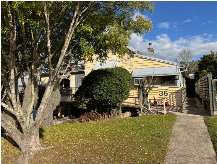
Figure 6 The dwelling at #36Myles Street.
